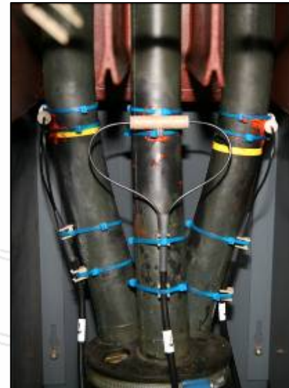
The DISCOS ® Sensor on the MV line
