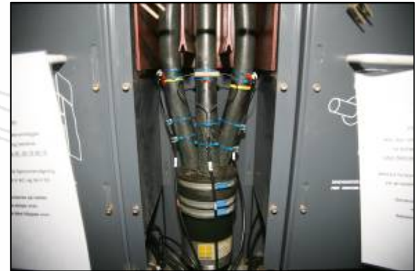
The DISCOS ® Sensor on the MV line
