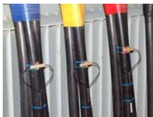
Figure 3, Installation of cable mounted optical sensors
